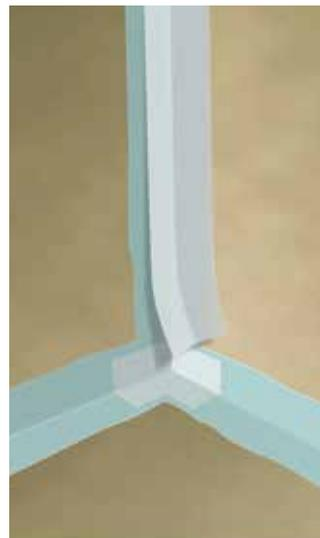
**STAGE 5** 2 coats of Tanking Paste should now be applied by brush, spatula or roller to all surfaces that require Tanking. Apply one coat horizontally and one coat vertically.
