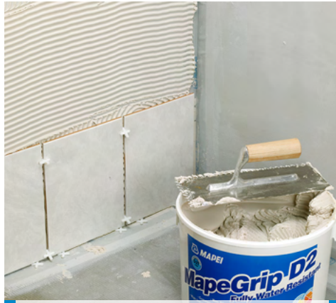
5. Tile using a suitable adhesive
