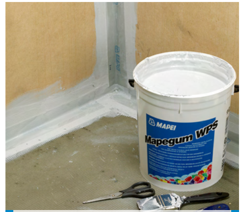
3. Apply the tape to the joints
