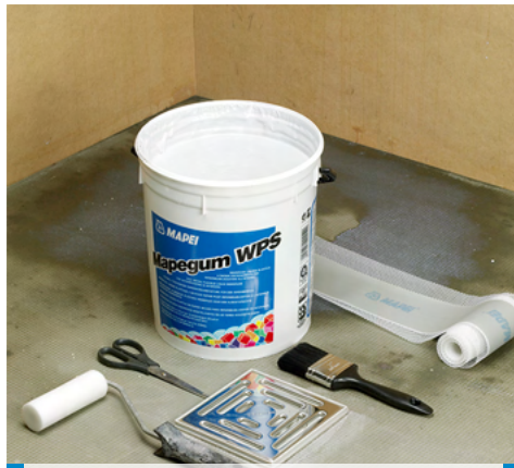
2. Prepare the tape for joints
